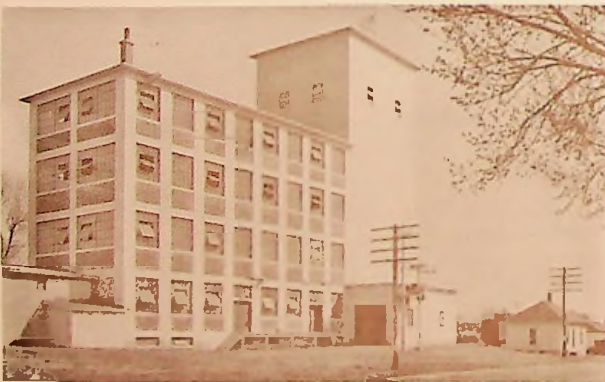
Gibbon Roller Mills constructed along the Union Pacific Railroad in Gibbon in 1919-1921.
