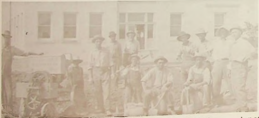
Hibberd Brick Co. and Keller Concrete Machinery Co. at work on the gymnasium at Kearney State Normal School, 1916. Richard Hibberd is the man with the beard in the back row in the center of the photo.
