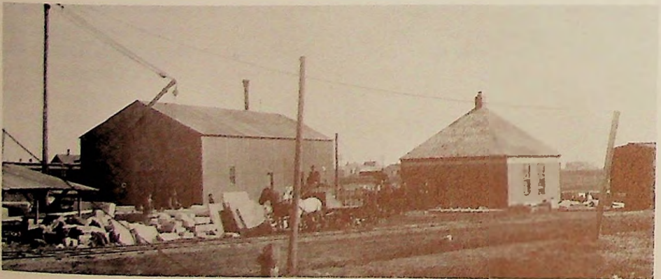
Kearney Stone Works, between Avenues B & C, south of Burlington railroad
