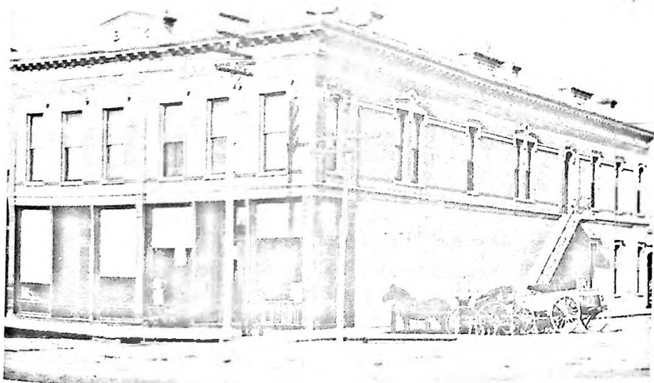
Switz Building, 1889, 2301-03 Central Avenue.
